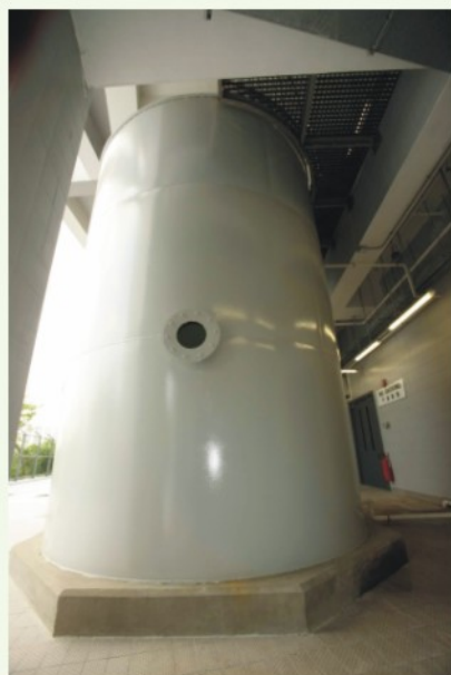
● 訓練水中切割焊接的直立式水缸 Welding Training Tank
